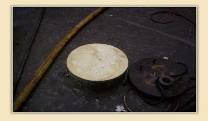
Foam is injected and allowed to rise in several continuous layers until the pontoon is completely filled. When full, any excess is trimmed from the manway. The **SINK-NOT 350** foam will expand into the smallest holes, sealing them against further leakage and corrosion.
