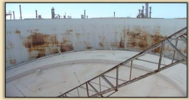
The above is an example of a sunken roof due to leaking pontoons. This is an all too frequent occurrence due to corrosion from rainwater above and product contact below resulting in:
